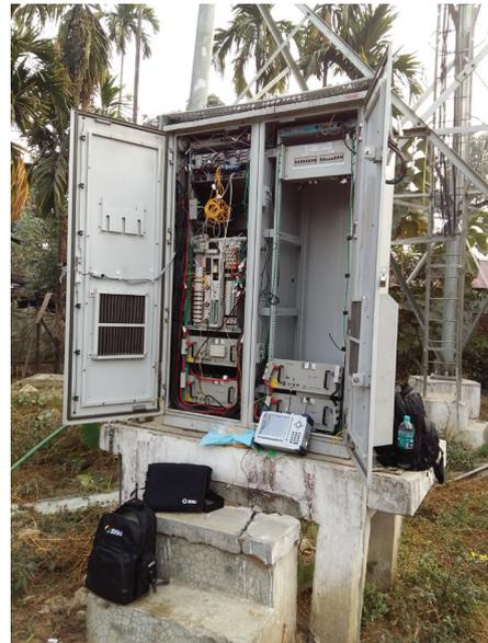
CellAdvisor tapping the BBU-RRH CPRI link — all measurements are at ground level
