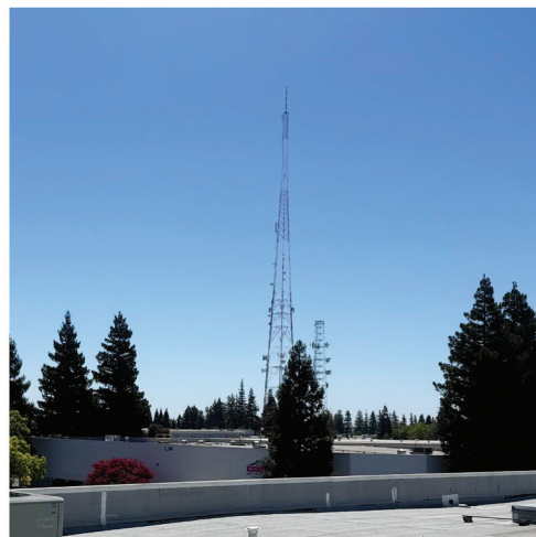
Cellular Communication Tower View from the Building Complex
