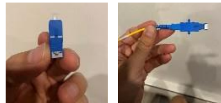
Figure 8: OTDR module connection to non-reflective termination
