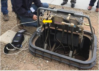
4. Connected off the seizure screw of the DC or Splitter with the leg showing the CPD
