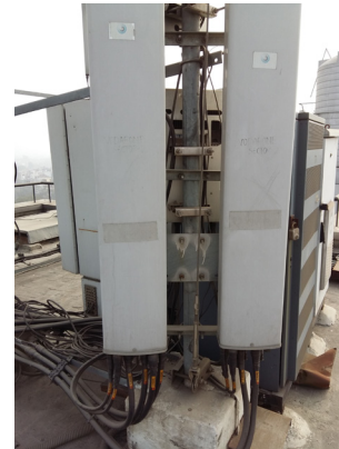
Figure 3: PIM generating antenna
