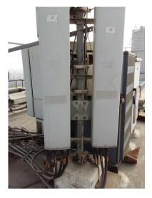
Figure 3: PIM generating antenna
